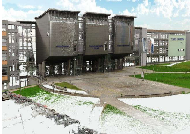
Figure 2 –Scanned object- Uniza ŽU after processing 5
