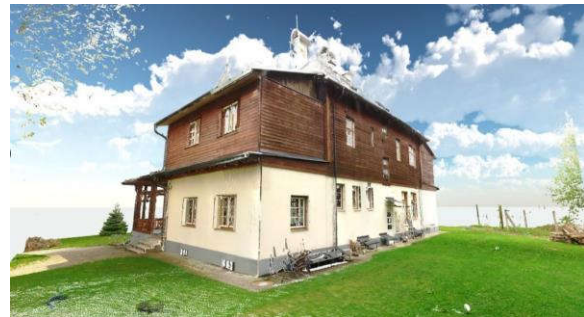
Figure 2 – Post-processed scan of building. Done by Laser Scanner
